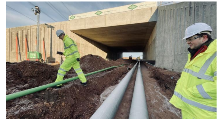
Heat pipe ducts laid under A1, Shawfair Project [Provided by Vattenfall 2023]
